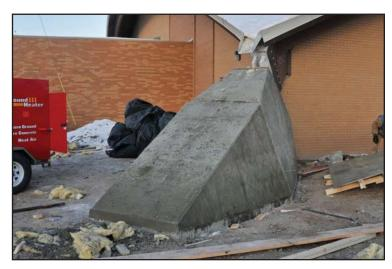
The rotted bases were replaced with a new hinge assembly and reinforced concrete. Similar repairs are planned for the southwest and northeast corners this spring.
